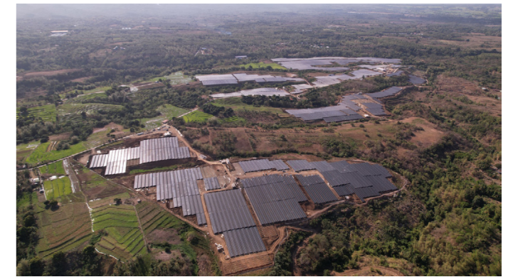
Prime Infra's solar power plants in Batangas and Cavite, to be commissioned in April 2024, have a combined supply capacity of 140 megawatts.
