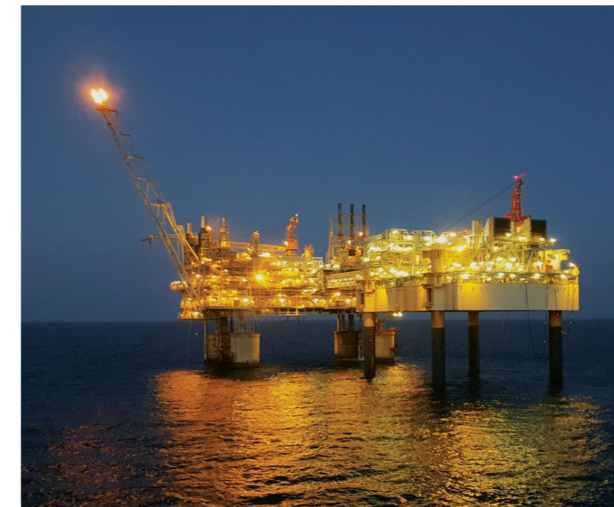
Prime Infra, through its subsidiary Prime Energy, is now in the process of Malampaya Phase 4 drilling with the aim to deliver new gas by 2026.
